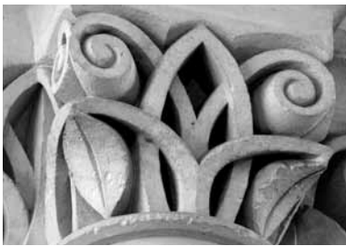
Cauffry crossing, replaced
